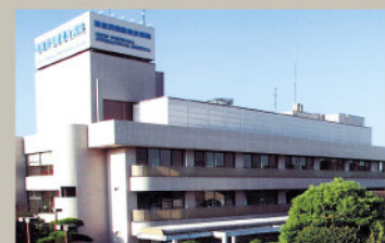
Nishi Yokohama International Hospital
